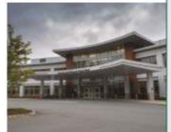
Dartmouth-Hitchcock Heater Road
